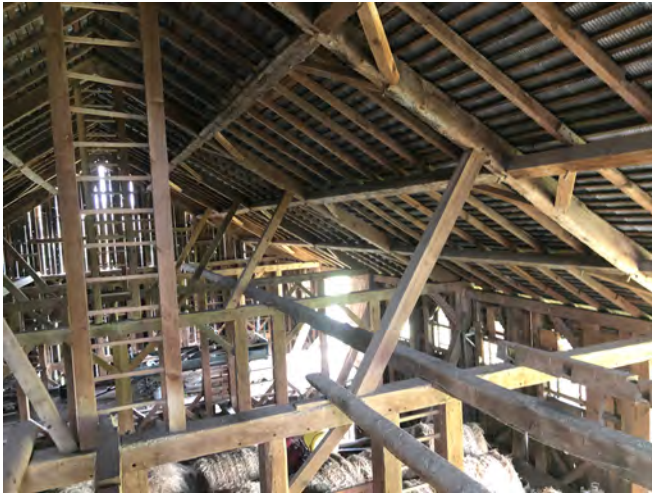
Exposed interior September 21, 2021
